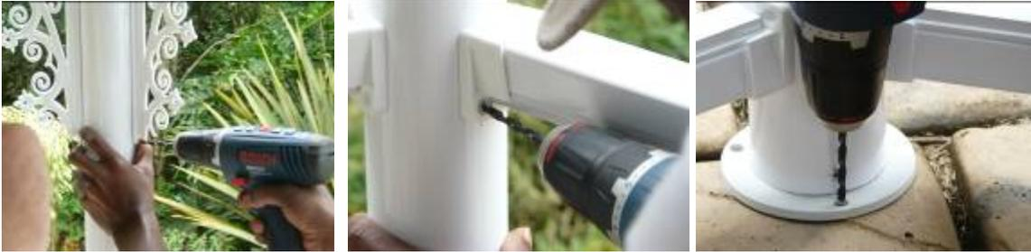
Finally, drill through the holes at the bottom of the post flange. Using anchor bolts or Any suitable bolts (not supplied), secure all posts to the the surface
