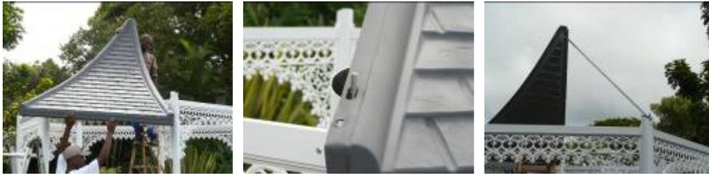
When the roof panel is safely secured onto the Support Pins , the second person should ,whilst holding the Support Bar, climb the ladder which has been placed in the centre of the gazebo, and place the fitted ring found on the end of the bar over the Roof Support Pin directly in front of the roof panel. The first roof panel is now held safely in place and one can continue to work with the other panels without fear of the first one falling.
